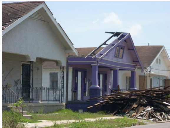
Photograph 5-3. Damaged houses in the study area.
