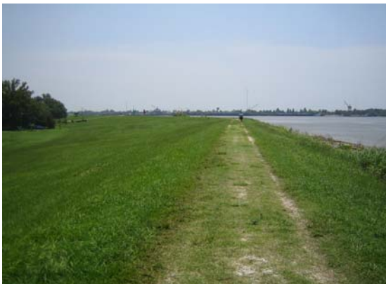
Photograph 5-8. Holy Cross levee with recreational trail.
