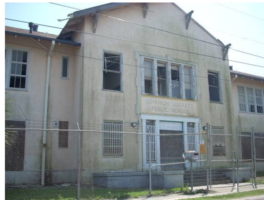
Photograph 5-2. Johnson Lockett Public School which has not reopened since Hurricane Katrina
